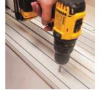
Pre-drilling bottom running track for screw fixing it on floor. Bottom running track should be offset from the front of door
