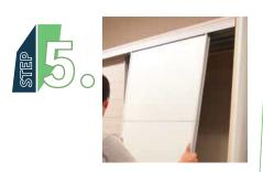
After installing top and bottom running tracks, insert door into top running track first then tap door bottom wheels until wheels are aligned with bottom track to put wheels in.
