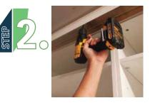
Pre-drilling top running track for screw fixing it to door jamb. Top running track should be flush with the front of door jamb.
