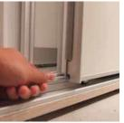
Adjust door bottom wheels with 4mm Allen key until door is leveled. Clock-wise to tighten and raise bottom wheel.
