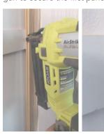
Secure with pin gun at female side before stacking next panel. Hammer the newly added wall panel to make sure it is fully inserted.
