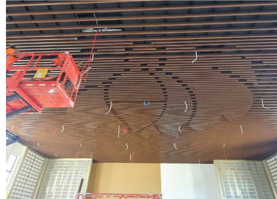
Suspended ceiling with lotus pattern during installation process
